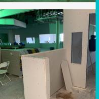
We now have the second side of drywall up in most of the spaces and HVAC is roughed in. Electric has been pulled and now we are getting ready for some fun stuff!
